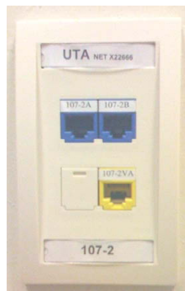
Photo 23: Picture of Proper Faceplate Configuration
