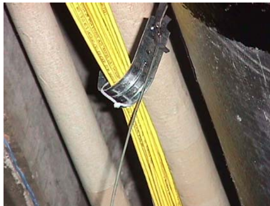
Photo 12: Proper use of CADDY J-Hooks.
