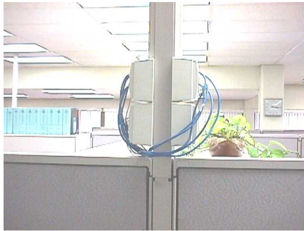
Photo 24: Example of single gang surface mount boxes with executive faceplates mounted on a power pole feeding top-caps.
