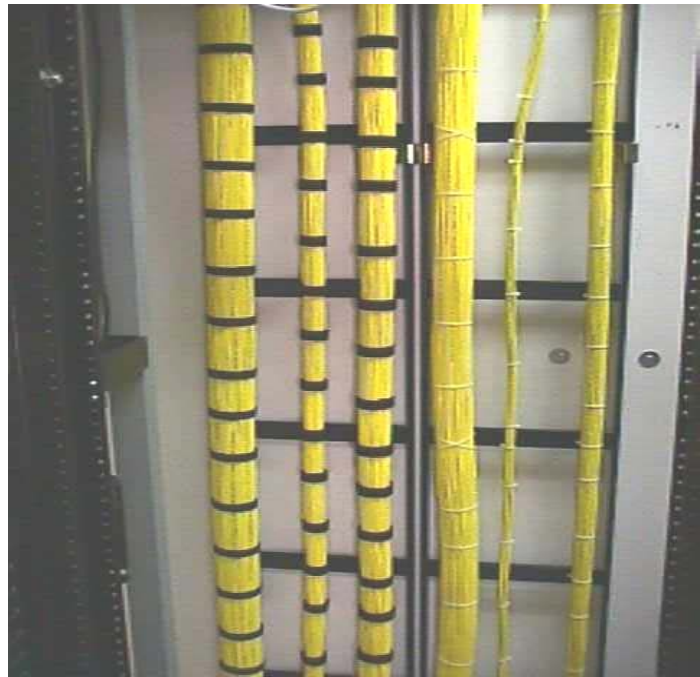
Photo 7. Proper transition between floors. Bundles are correctly secured to vertical ladder sections by cable ties or Velcro straps.
