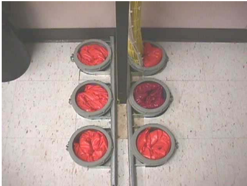
Photo 35: Properly Fire-stopped using SpecSeal™ Intumescent Pillows
