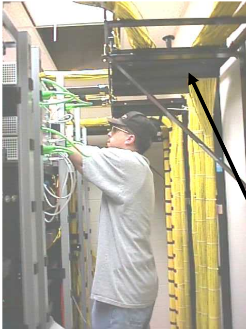
Photo 6. Proper use of waterfall (rounded transition) fittings for cable changing from a horizontal path to a vertical one. This maintains the minimum bend radius for Cat 5e/6 cable.
