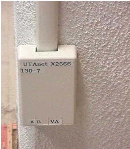
Photo 21: Example of 4-port PANDUIT surface mount box (P/N CBX4IW-AY).
